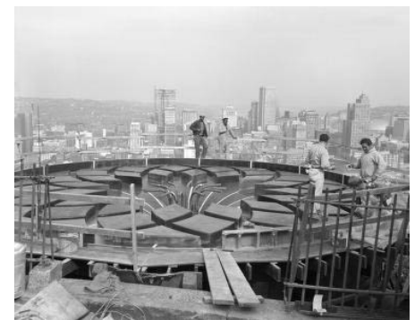
Construction of an overlook in 1967
