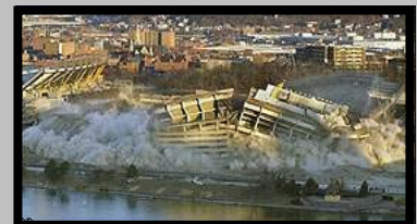
A view from Mount Washington of the demolition of Three Rivers Stadium
