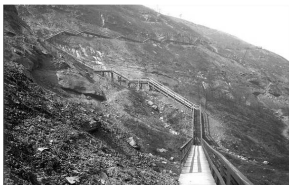
Image 4 View of the former 'Indian Trail' stairs climbing the face of the mountain.
