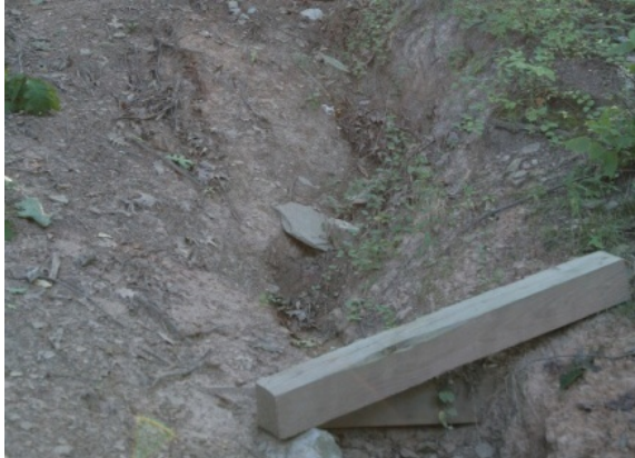
Image 15 Severe erosion, typical along some trails in the Mount Washington Park area.
