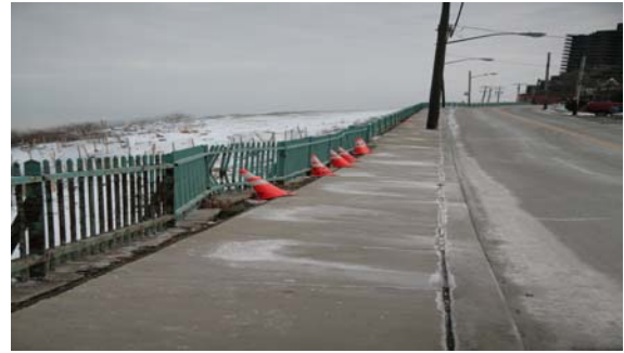
Image 11 Sidewalk and railing condition along Grandview Avenue at the terminus of Shaler Street.
