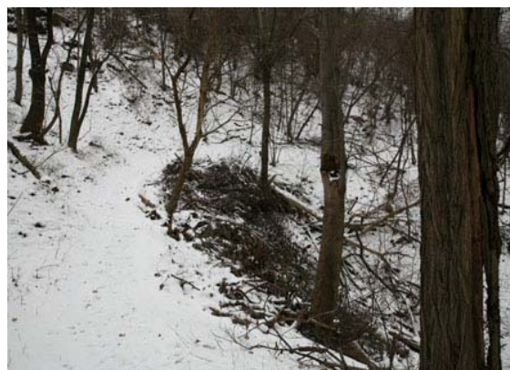
Image 7 Brush debris placed along the trail in Grandview Park in an attempt to stabilize the slope.
